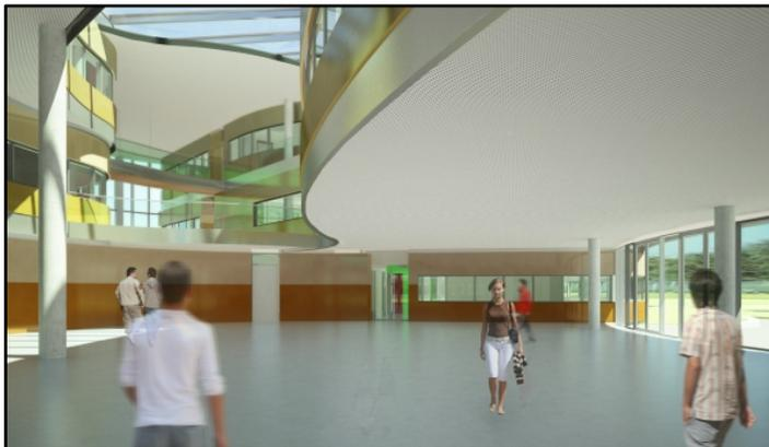
The positive point of the flexibility is the application of lightweight partition walls and the column free aula in the centre of the building. This makes it possible to change the form of the rooms, as far as possible because of the column structure.
