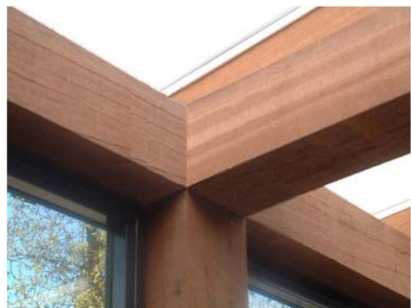
Figure 2 Desired joint without connection material
