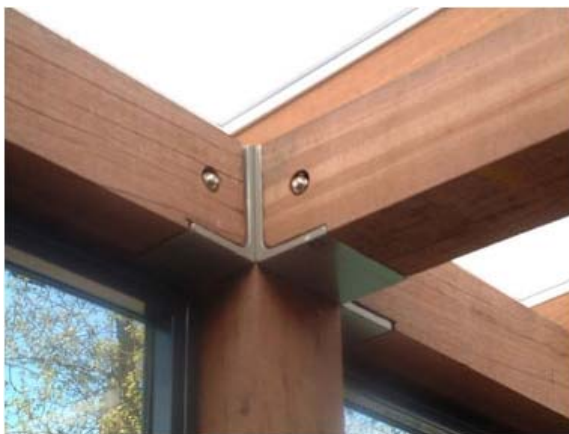
Figure 1 Joint with connection material
